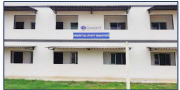
Building Units planned and executed using Glass Fibre Reinforced Gypsum (GFRG) Panels by Faculty and Students of Civil Engineering Department
