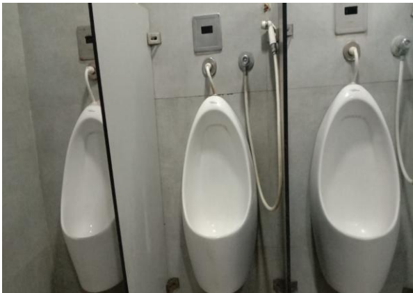
TOILET FLUSHING WITH REUSE WATER –DUAL PLUMBING
