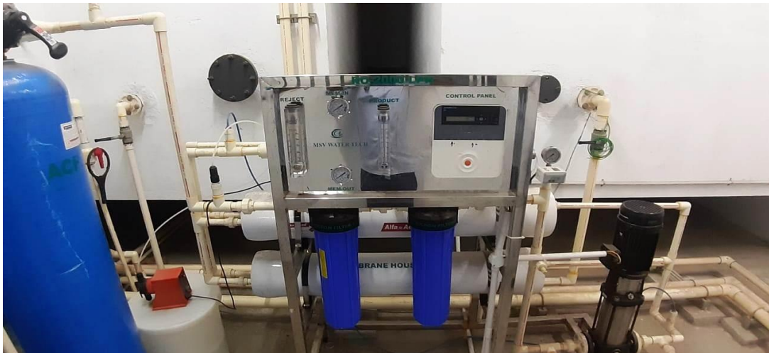
ARCHITECTURE BLOCK RO PLANT
