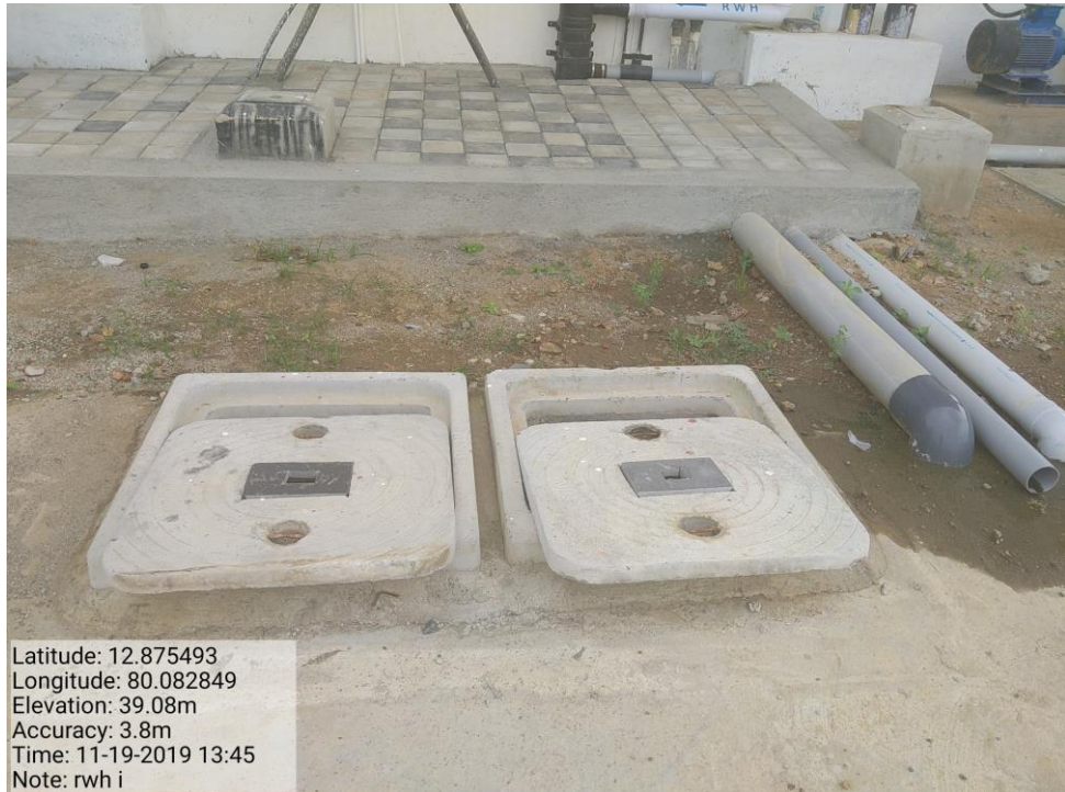
RAINWATER COLLECTION SUMP (ARCHITECTURAL BLOCK)
