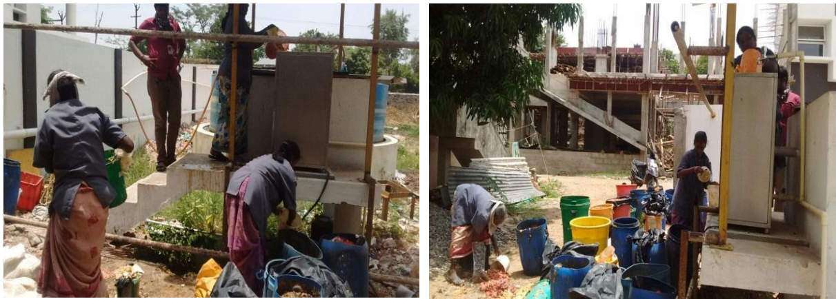
Food waste feed in to Bio Gas Plant
