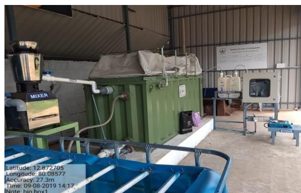
BIOBOX- Biogas generation unit
