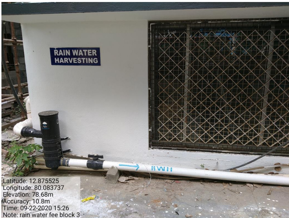
RAINWATER COLLECTION SUMP (ARCHITECTURAL BLOCK)
