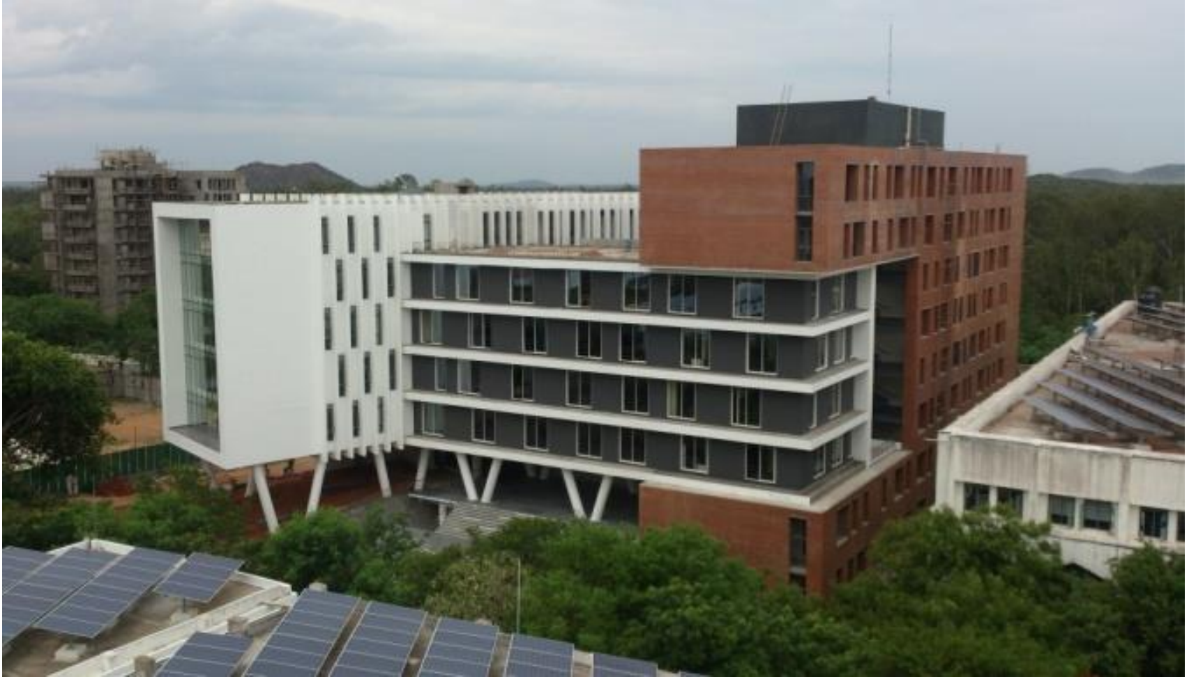
School of Mechanical Sciences Building (2014)
