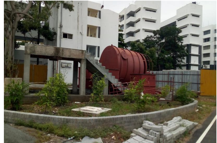
Installation Work in Progress
