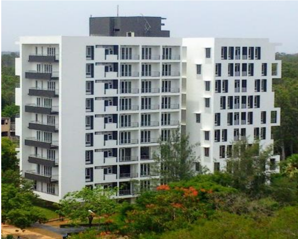
New Staff Quarters (2015) Built up Area: 75000 sft. (G+9) Project Cost: Rs. 17 Crores
