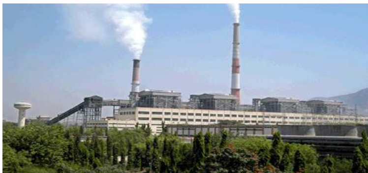
Figure 1.1 Mettur Thermal Power Plant
