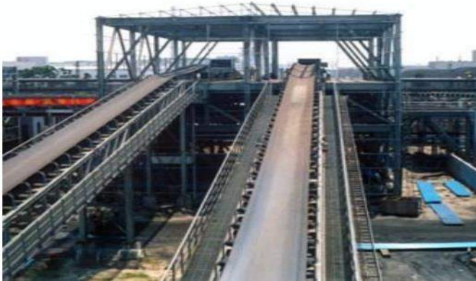
Figure 2.2 Coal Handling Plant –Coal Mill
